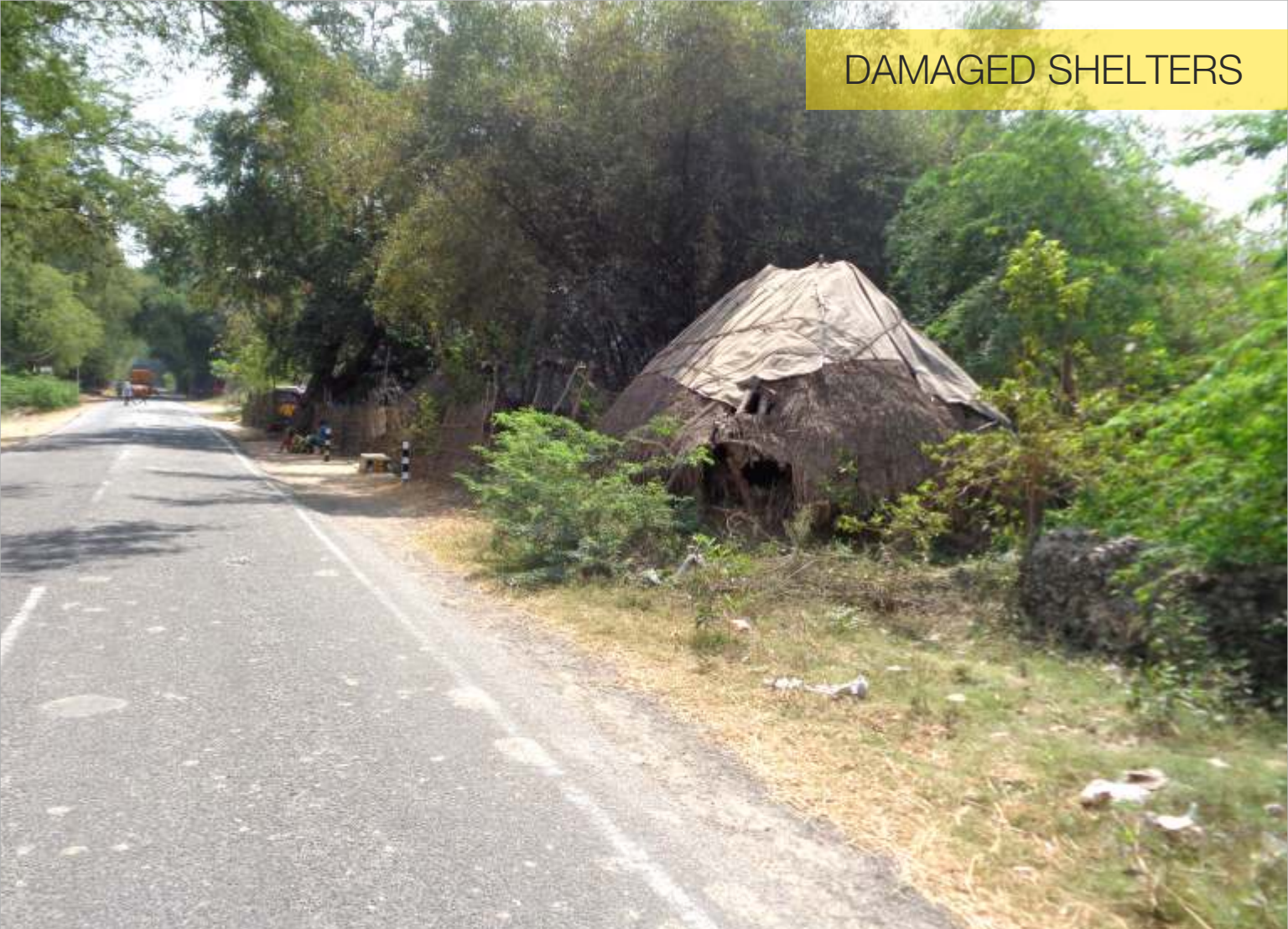
C. Sathamangalam 2 - 43 Houses
