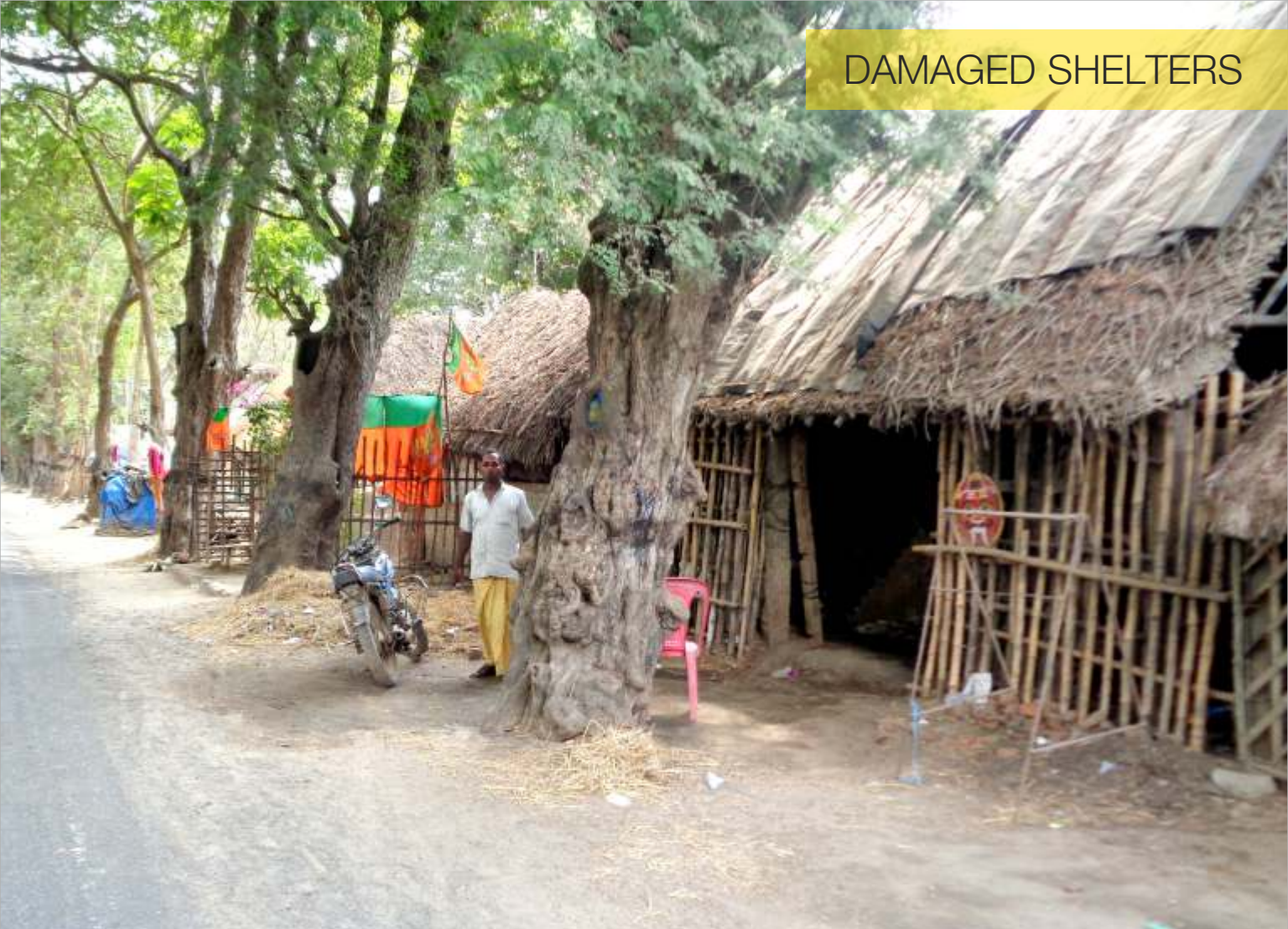
C. Sathamangalam 1 - 22 Houses
