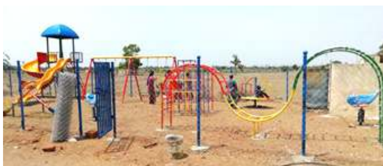
Classroom And Playground Renovation, Elementary School, Kovilur
