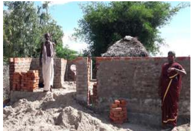
Cyclone Gaja Relief Project, Pannaiipothu
